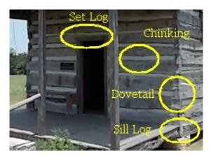
Above are some of the terms used in the construction of a log cabin.
